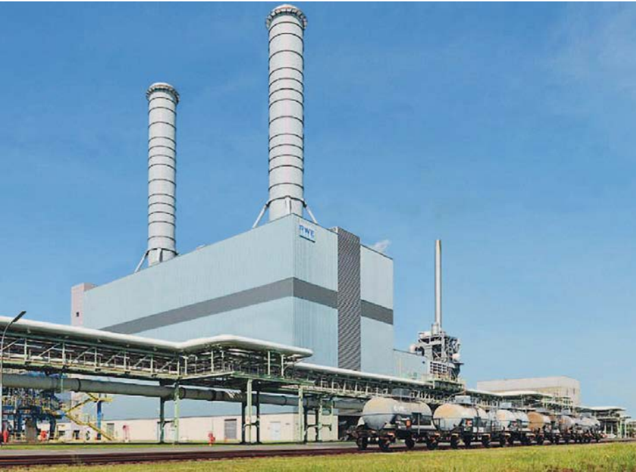
Dormagen combined cycle plant
