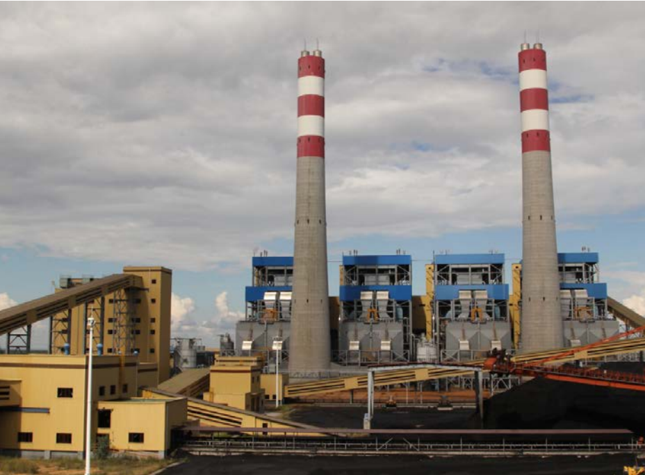
Morupule B coal-fired CFB Power Plant in Palapye, Botswana
